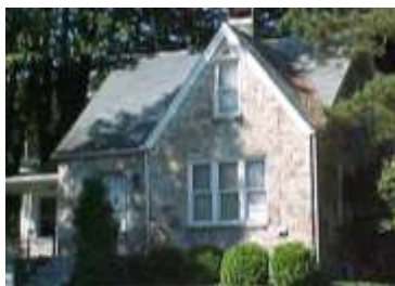
Sutton/Ulrich Cottage, Mahaffey Camp and Conference Center, Mahaffey, PA
